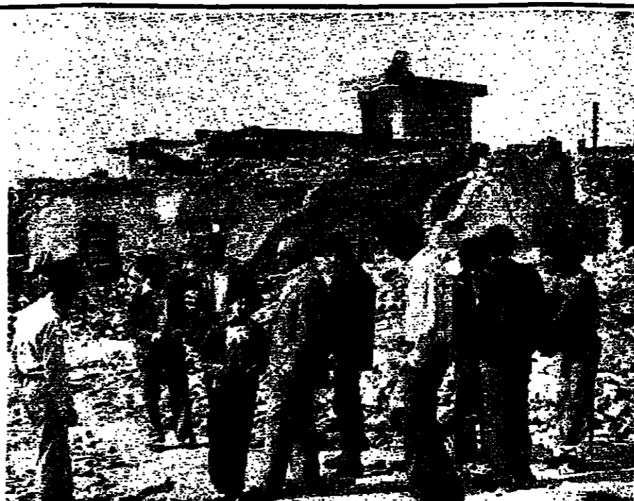
ASSESSING DAMAGE: Relief volunteers inspect damage in Dezful caused by Iraqi missile attacks recently.
